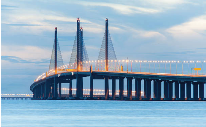
Figure 1.10: Penang Bridge (Credit: Lee Chee Keong)
